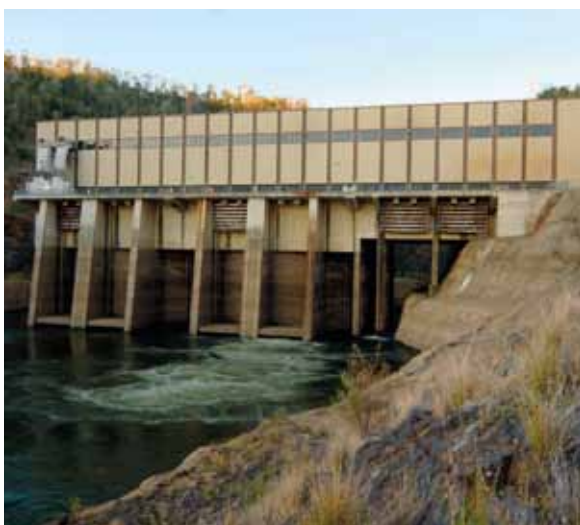
Pumped hydropower is an established energy storage technology that can be used with all energy sources for provision of on-demand power, here used at Wivenhoe Power Station in Queensland. Source: CS Energy
