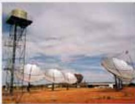
**Concentrated solar PV:** Lenses or curved mirrors are used to concentrate a large amount of sunlight onto solar photovoltaic cells. These systems can be more efficient than regular solar PV, since less photovoltaic material is required to produce the same amount of power. Tracking systems are also used with concentrated and regular solar PV, to follow the path of the sun through the day and maximise the amount of power produced.
